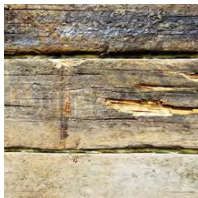
FACADE upper part
